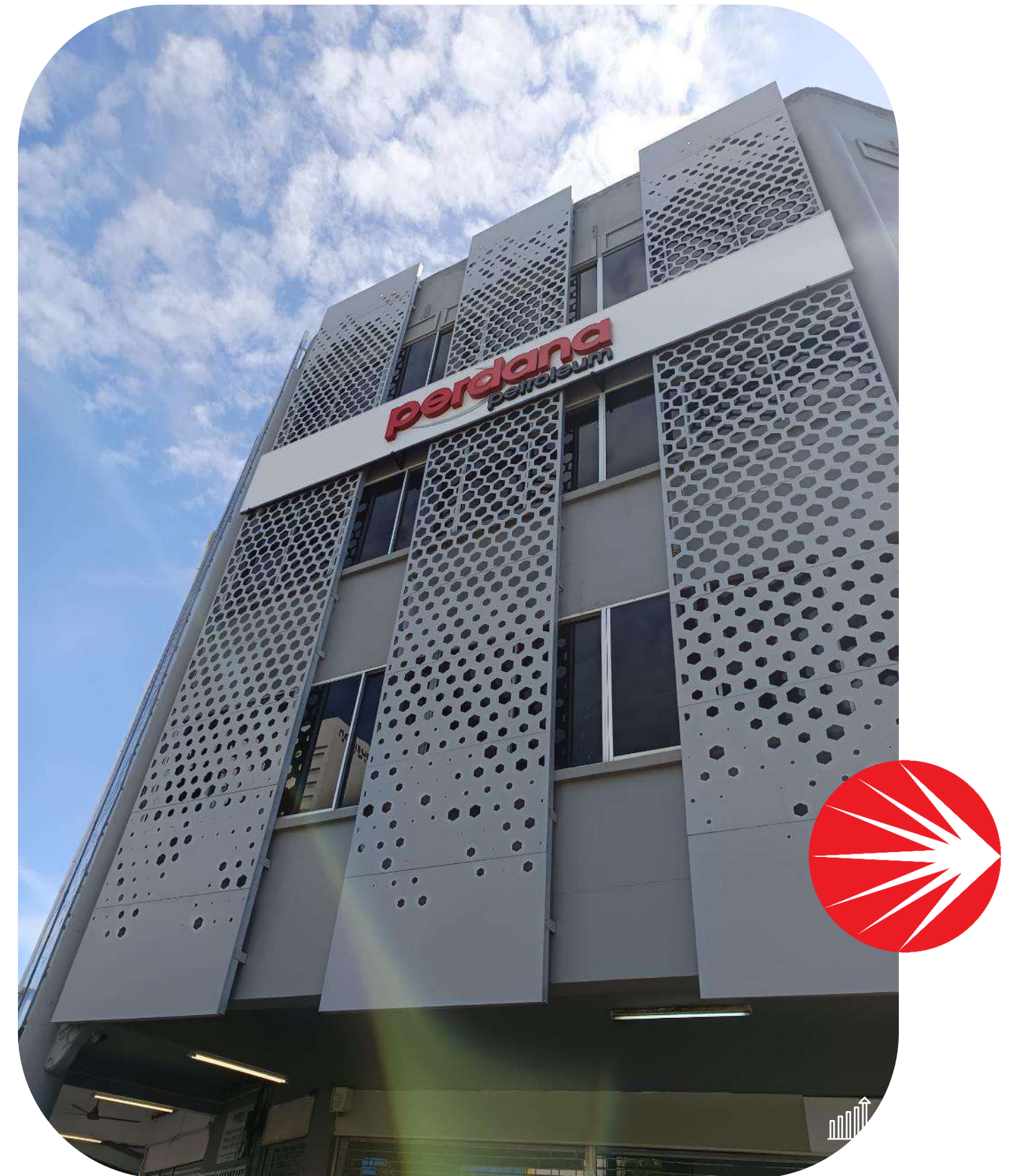
Miri Office (Shoplot Premises)
